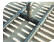
Collectors Arms Internal Distribution System
